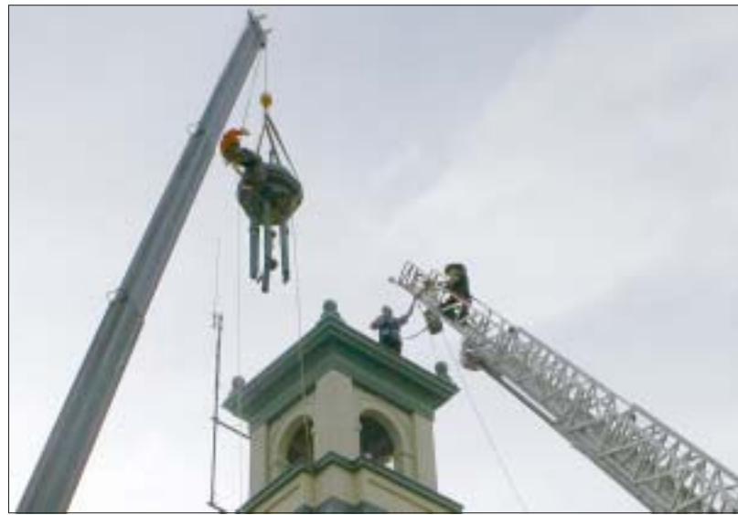
EASY DOES IT (May 11)...Workers carefully remove the spire atop of the Westfield Fire Headquarters after painters reported safety concerns.
