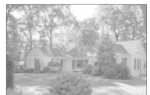
Burgdorff ERA Realtors, 600 North Avenue West, Westfield is pleased to announce the sale of 2659 Fairview Drive, Scotch Plains. The selling agent was Grace Rappa.
