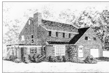
Century 21 Taylor & Love, Inc., 436 South Avenue, Westfield has announced the sale of the above property at 722 Knollwood Terrace, Westfield. The property was marketed by Barbara Doherty.
